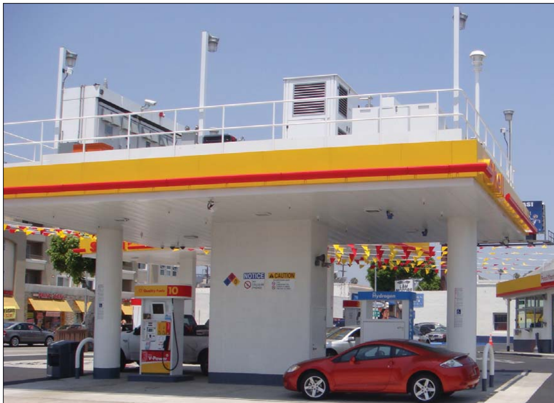
At a Shell retail gas-hydrogen station in West Los Angeles, hydrogen fuel is produced on site by an electrolyzer on top of the station canopy. Photo from Photographic Services, Shell International Ltd.
